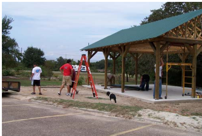
(Omega Delta Phi helps with laying the metal roof.)
